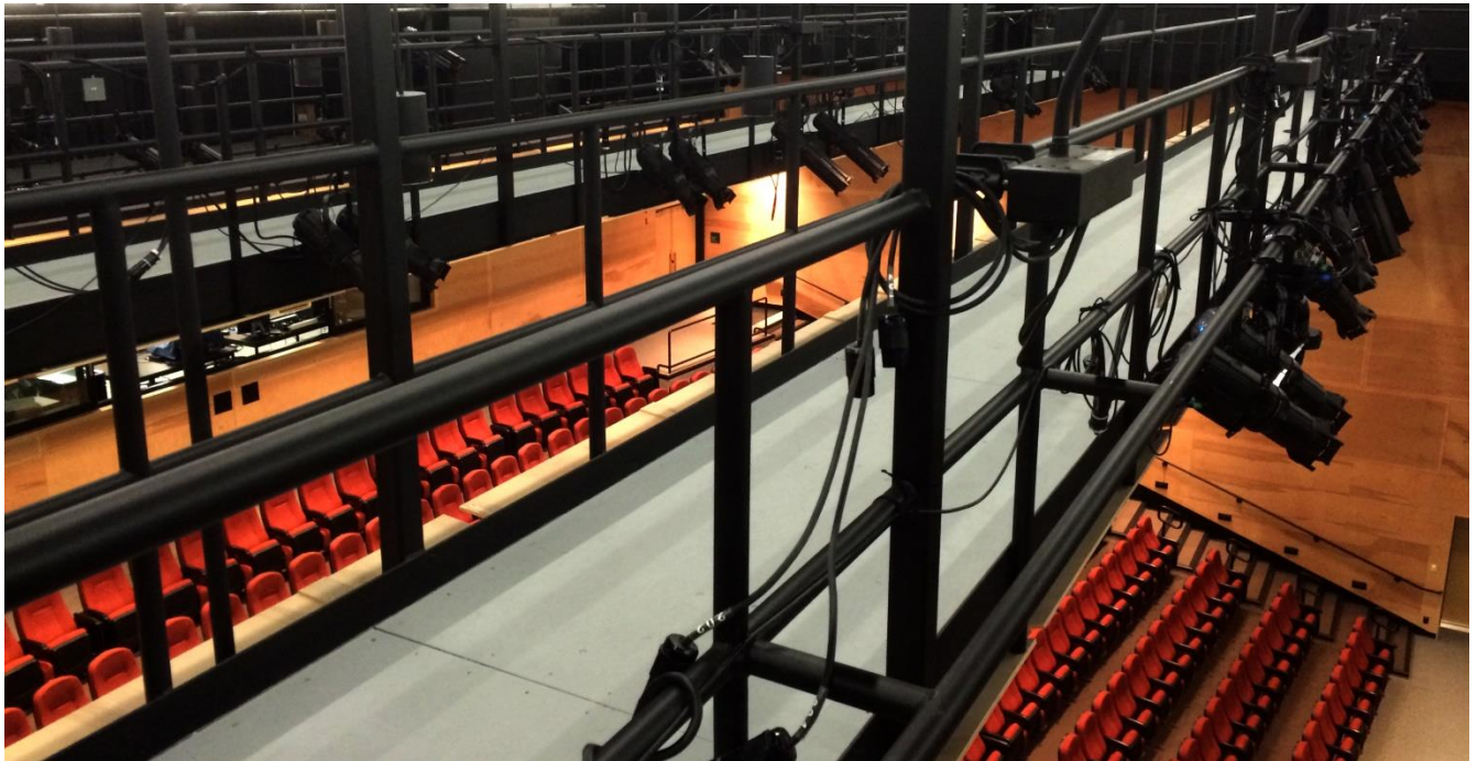
Figure 7 – Catwalk access to lighting fixtures above the seating area
